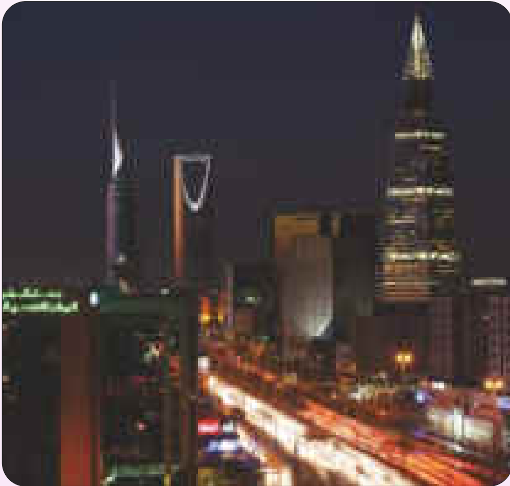
(Kingdom Tower, Riyadh)
